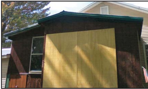
Image 8. Was there missing insulation here?
